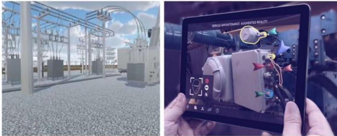
Figure 3: BIM integration with VR (left) and AR (right) technologies for a substation project.
