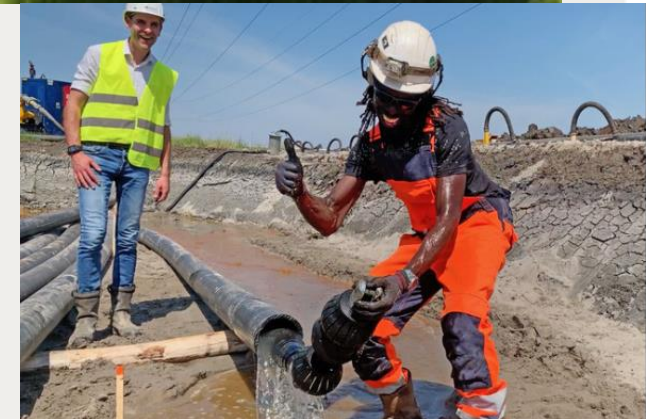
Water floating installation
