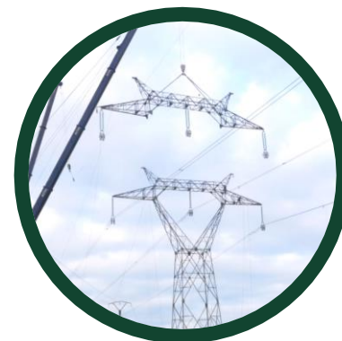
Live Line Working with cranes
