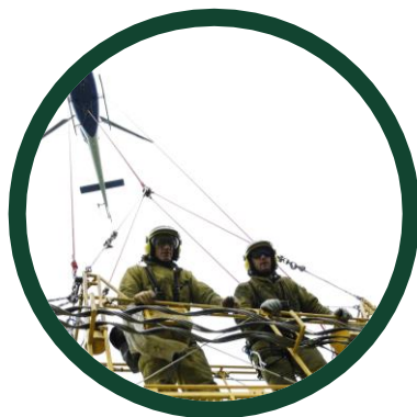
Live Line Working with a Helicopter
