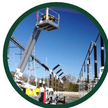
Live Working in Substation with an insulated Elevating platform
