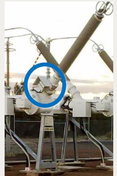
Electronic IT and process bus in 'digital' station
