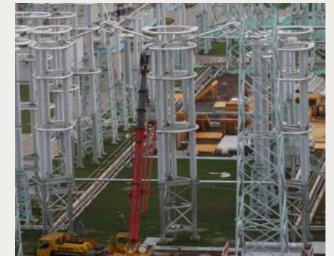
800 kV DC disconnector
