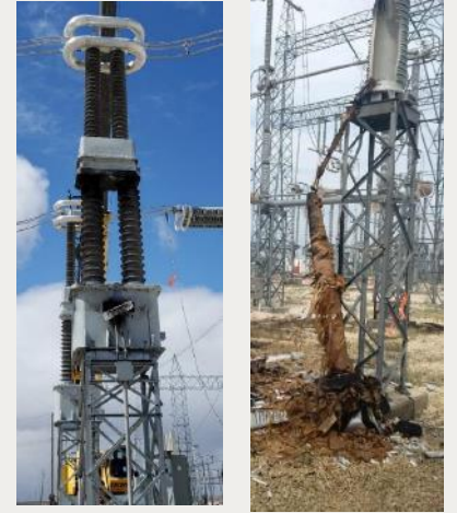
600 kV CT, dry, oil-filled after IA
