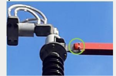
Temperature sensor in DS blade
