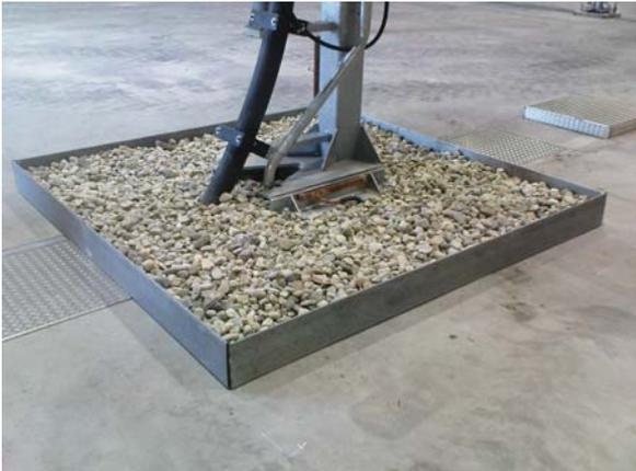
Figure 3: Grit-bed under a 380 kV cable termination to prevent spreading burning oil.
